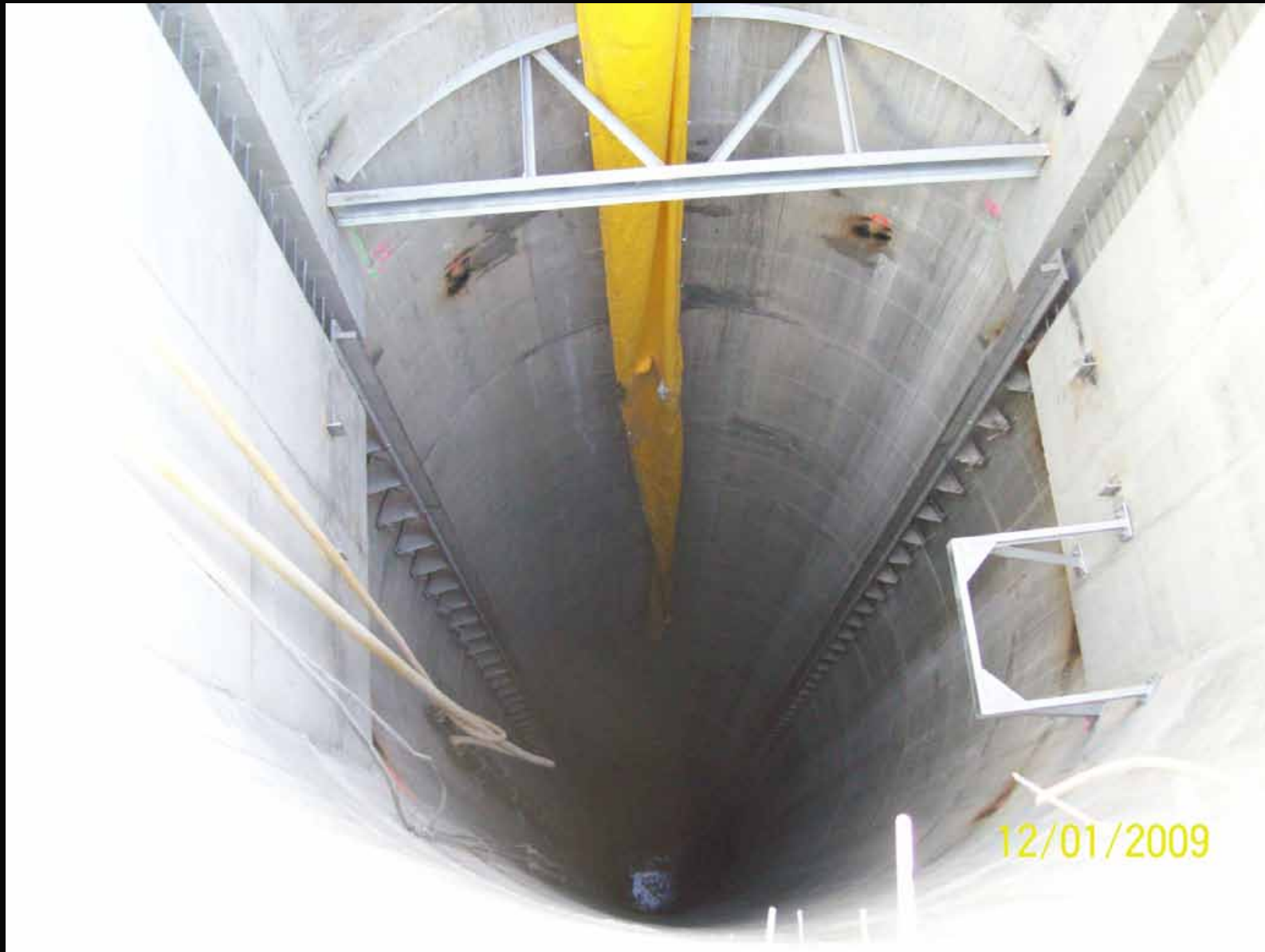
Gate Guide Rails – Stainless Steel
