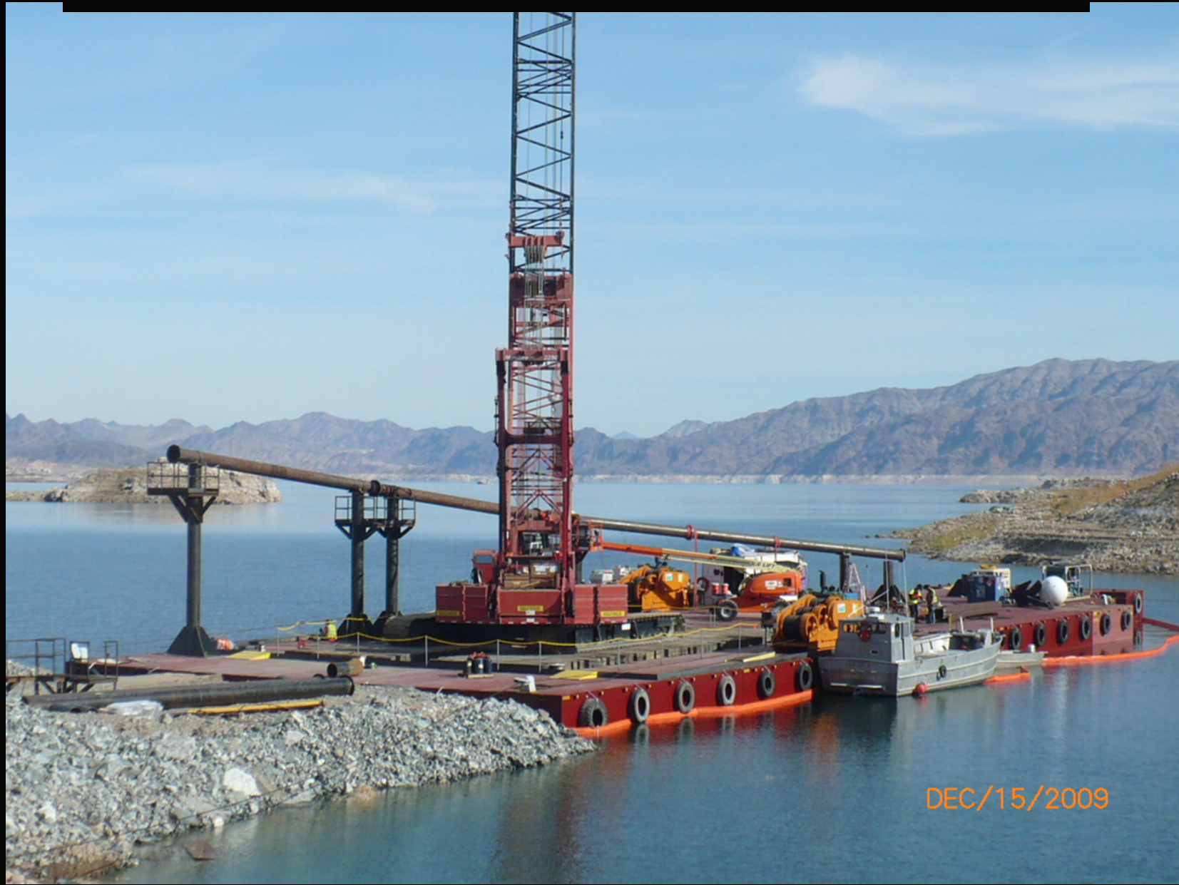
Crane/Excavation Barge – Dredging Pipe
