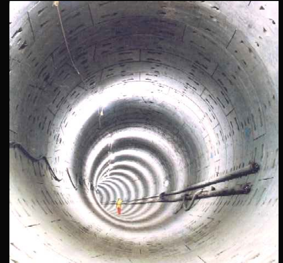
Precast concrete segmental lining
