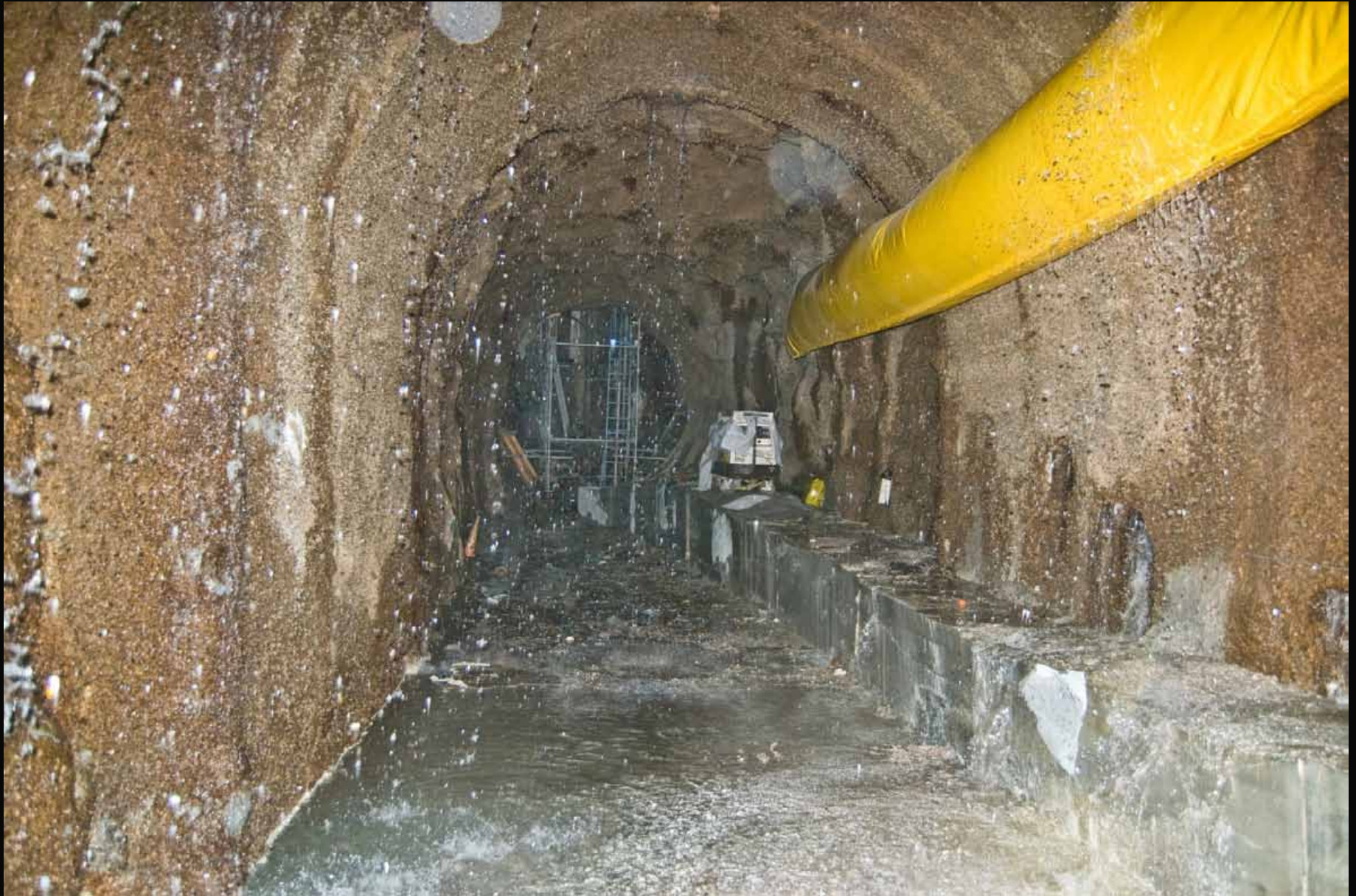
Intake No. 2 – Dewatered Tunnel (~ 1000 gpm inflow)
